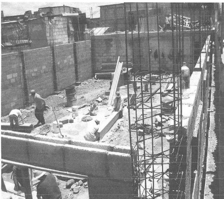
Construction of the walls and columns is nearly complete
